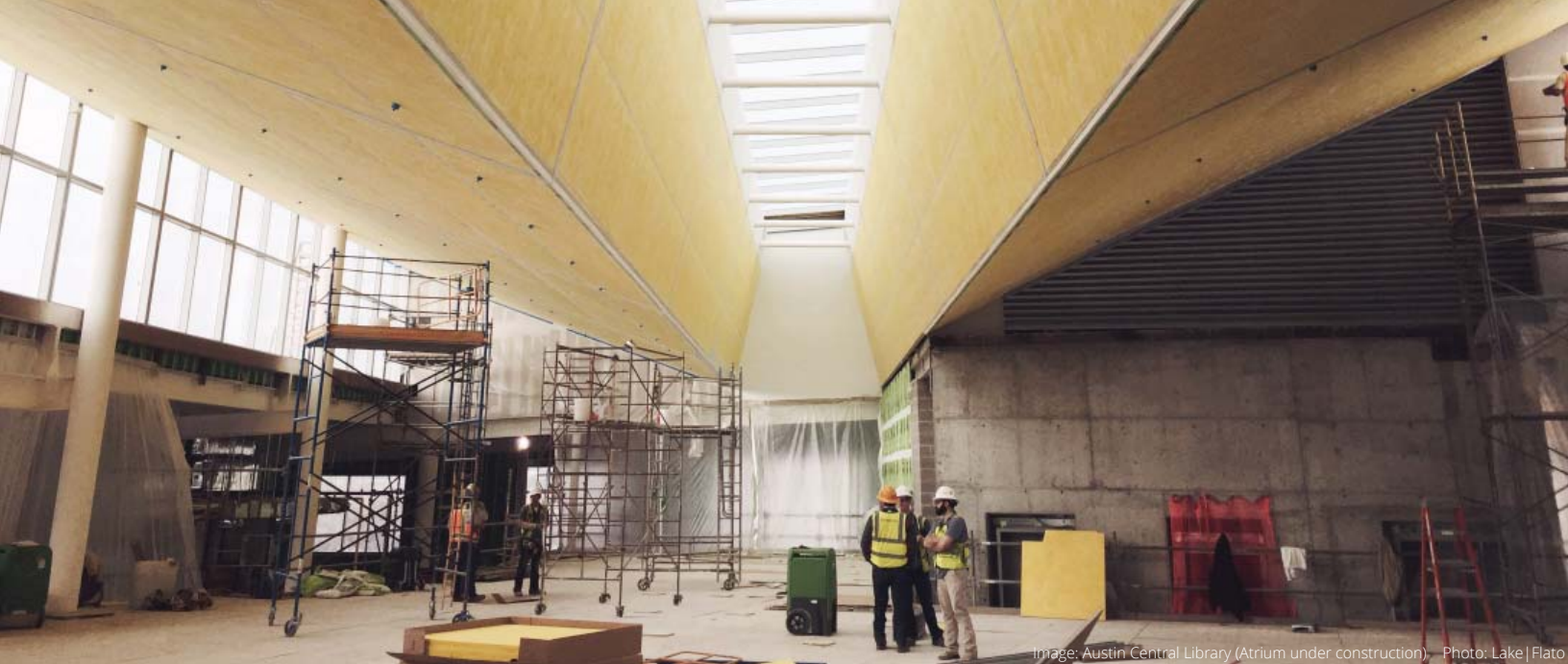
Image: Austin Central Library (Atrium under construction). Photo: Lake | Flato
